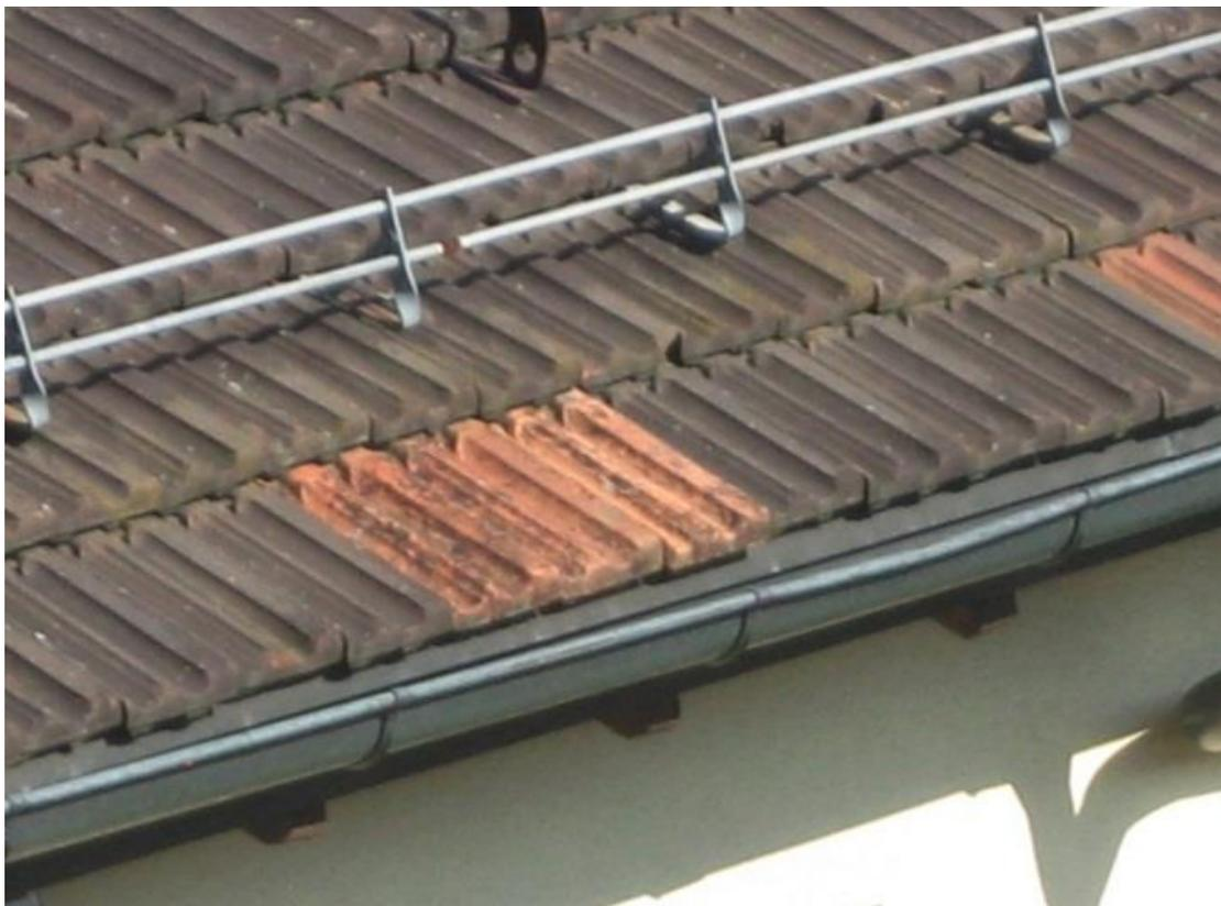
**Figure 12:** Weathered and replaced bricks on a roof
