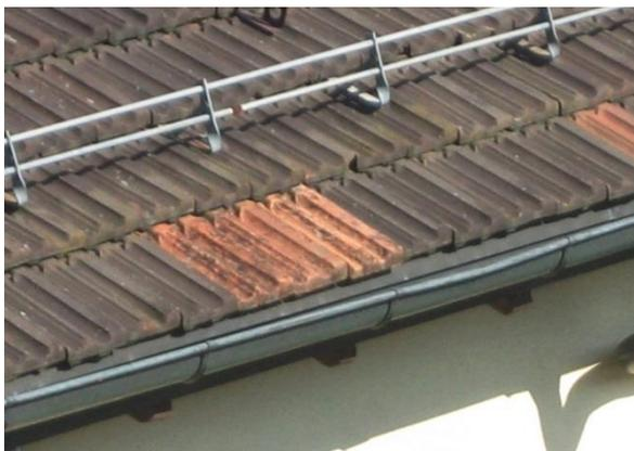
**Picture 1:** Aged roof with separate newish bricks
